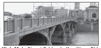
High-Main Street Bridge in Hamilton, Ohio
