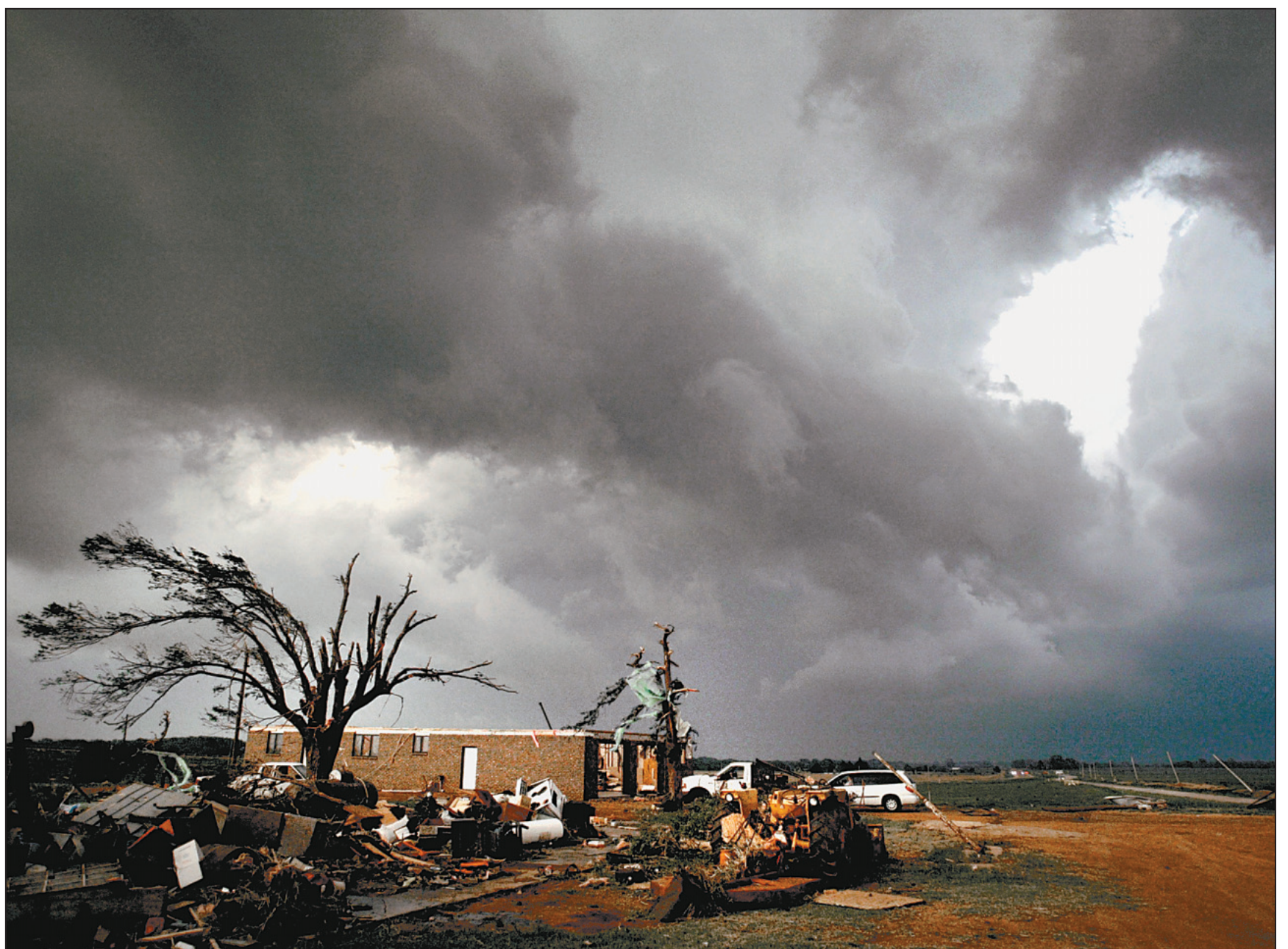
A home on the outskirts of Attica, Kan., lies in ruins — destroyed by a tornado — as more storms move in during search and rescue operations.
